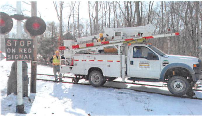
BT-1 with a crossing gate at Winkler Road
