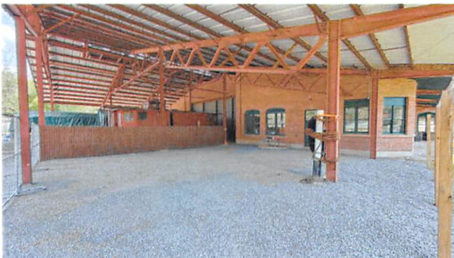
Train Shed Clean Up Results
