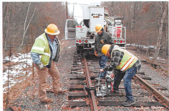
Repairing Winterfest Bonds with the Rail Drill
