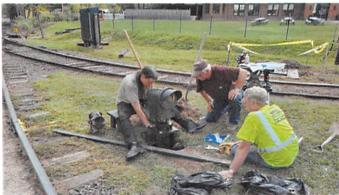
Dwarf Signal Repair at North Road Interlocking
