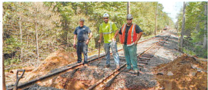
Replacing the Failed Culvert between Station 7 & 8
