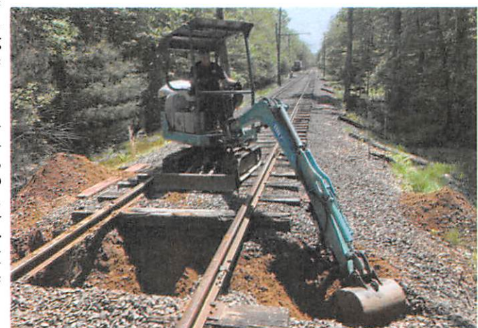
Replacing the Failed Culvert between Station 7 & 8
