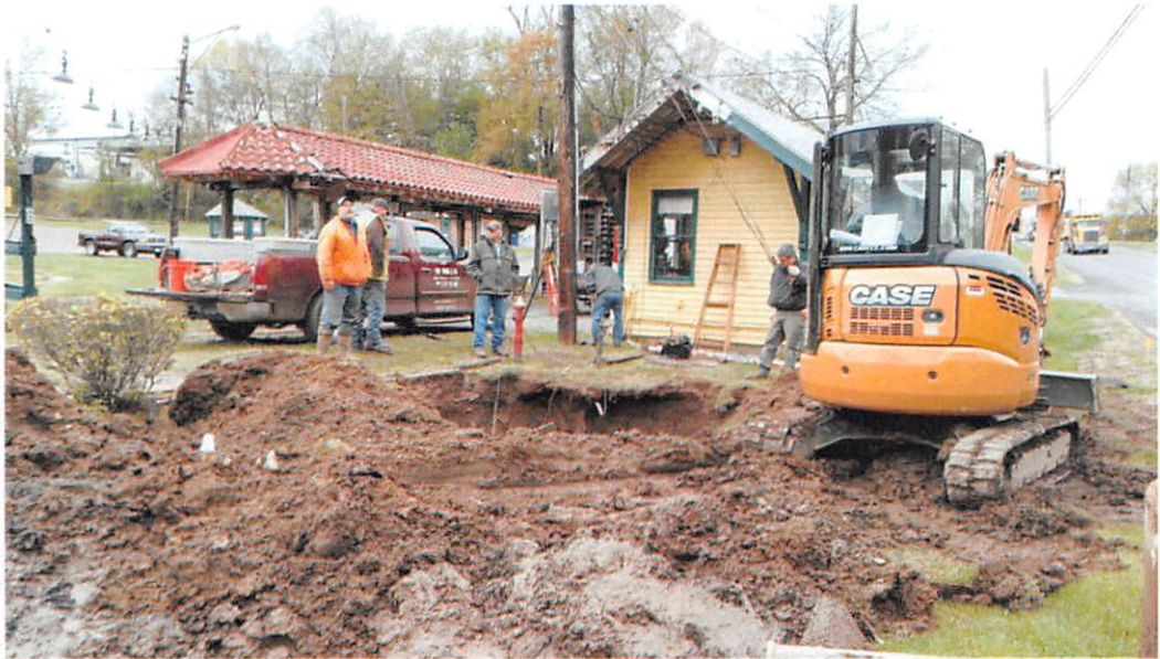
Replacing the Water Meter Pit
