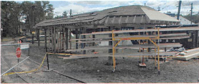
Isle of Safety During Restoration
