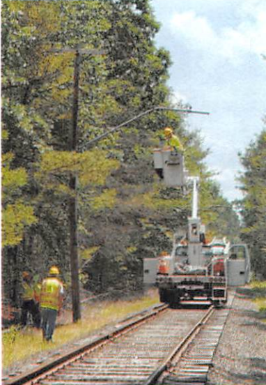
Repairing Overhead with BT1
