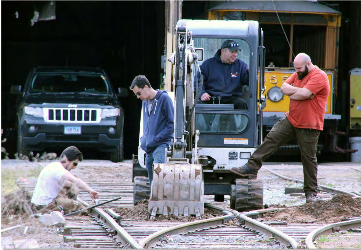
(L to R) Track Superintendent Dave Coppola, Ryan Boucher, Jake Foley and John Cummings replacing ties in Kelly Yard on March 26, 2016.
