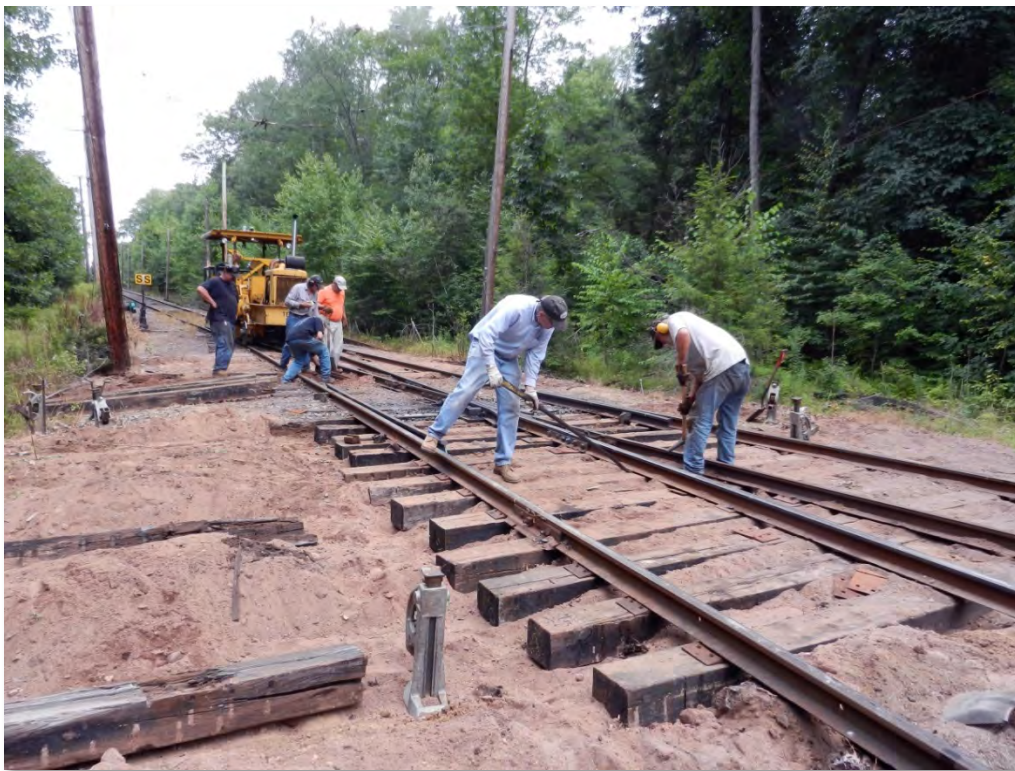
Mike Brenner (Center) working with the A. J. Belliveau crew replacing timbers at the East End of Hancock siding.
